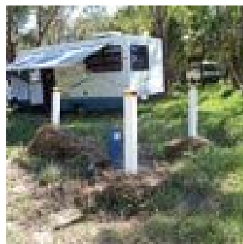
Debris against poles
